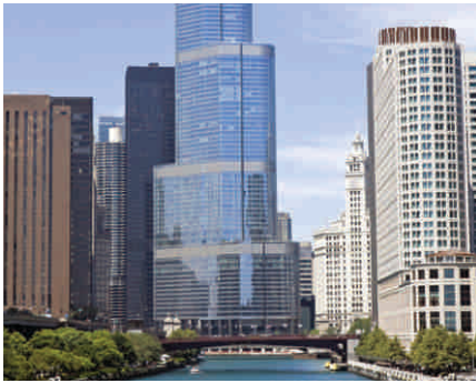
Trump Tower, Chicago, USA
